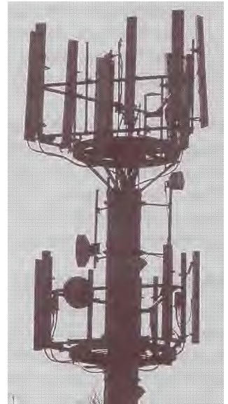
Figure 237: This little lot is right next to a public swimming pool and sports centre
