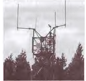
Figure 232: A TETRA mast
