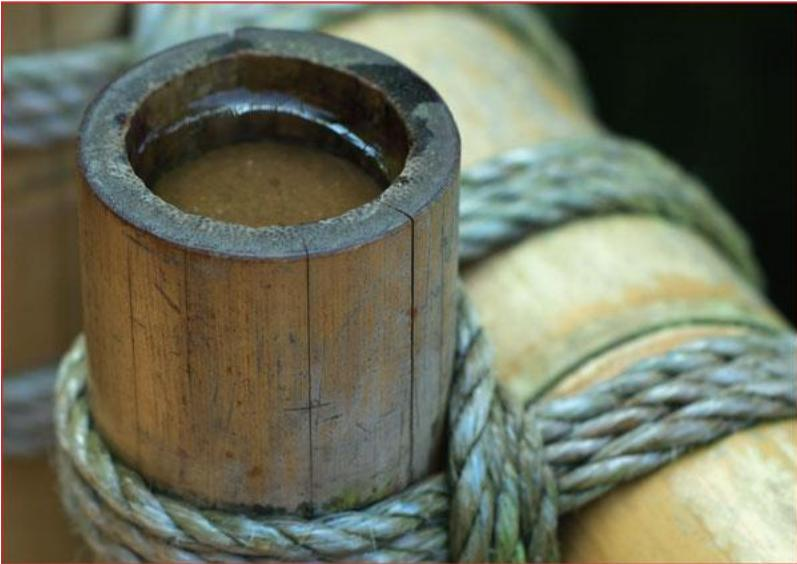
▲ A bamboo fence or gate can be constructed by lashing the bamboo together with strong rope.
