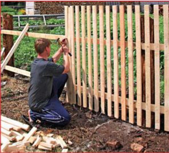
▲ A picket fence is constructed by nailing two or more long boards to posts, and then nailing narrow vertical boards to the horizontal ones.
