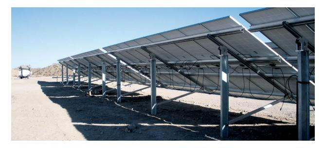
ABOVE: Standard ground-mount, single-post, cantilever design
