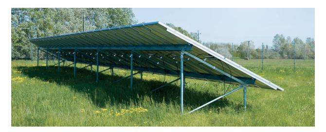
ABOVE: Standard ground-mount with two rows of vertical posts
