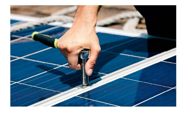
**3. Continue down the row.** Install more modules in the row, using the same techniques and adding WEEBs as needed. Check the
