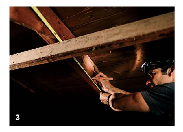
4. Locate the remaining rafters. Measure across the rafters for each remaining row, noting the locations of the anchoring rafters, as before. It's necessary to measure each row because the rafters may not be perfectly parallel to one another and/or each rafter may not be straight.
