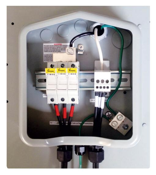
ABOVE: Box enclosures can function as junction or combiner boxes, in addition to anchoring conduit and making a watertight roof penetration. Locating a box under the array makes for a very clean installation; just be aware that you have to remove a module (or leave one off during the installation) to access the box.
