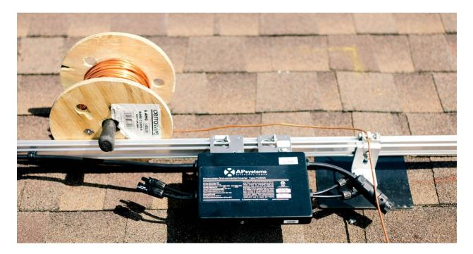
ABOVE: Microinverters typically are mounted to the racking underneath the modules. This microinverter connects to two modules. The heavier cables connect the microinverters together.
