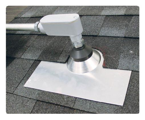
ABOVE: Standard penetration fittings include metal flashing and a rubber boot that seals around the conduit. High-quality fittings have a seamless metal cone at the base so that the rubber seal sits above the roof level to reduce wear.
