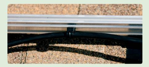
ABOVE: Rail clips (typically supplied by racking or microinverter manufacturer) fasten directly to rails.
