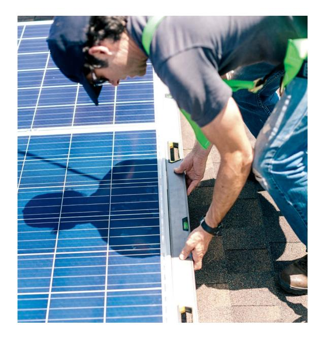
4. Complete the row. Secure the outside module at each end of the row with a pair of end clamps, using WEEBs, as applicable. Retorque all of the clamps in the row. Note: Remember to call for your rough inspection at the specified time, based on what the inspector wants to see of the modules and racking.
