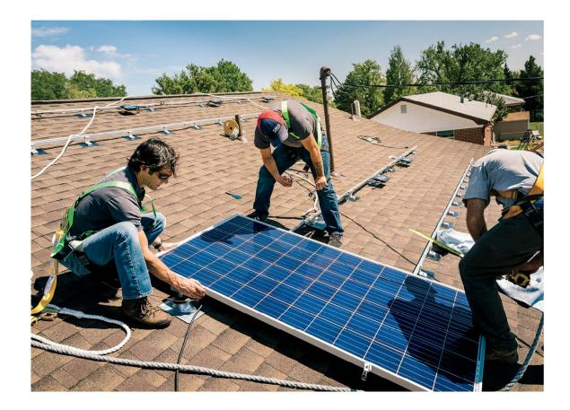
2. Position the second module. Set the second module into place and snug it up against the first module with the mid clamps (with WEEBs, as applicable) in between. Align the bottom edges of the first two modules, using a 4- or 6-foot level (simply as a straightedge, not as a level). Secure both modules with the mid clamps, and torque the clamp bolts as specified by the manufacturer. Connect the wiring as applicable.
