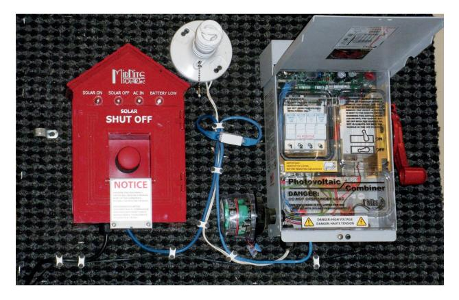
ABOVE: This demonstration setup shows a Birdhouse rapidshutdown control box next to a disconnecting combiner box. The blue wires are Cat-5 cables, which transmit the trip signal between the control box and the disconnect.
