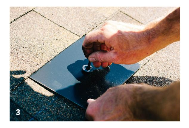
**4. Mount the footers.** Position each footer and footer base (as applicable) over a flashing piece and secure them with a lag screw through the hole in the flashing and into the pilot hole in the roof. If the footer can be adjusted on its base, leave it a little loose so you can move it as needed when positioning the rails (you will tighten the lag screws later).
