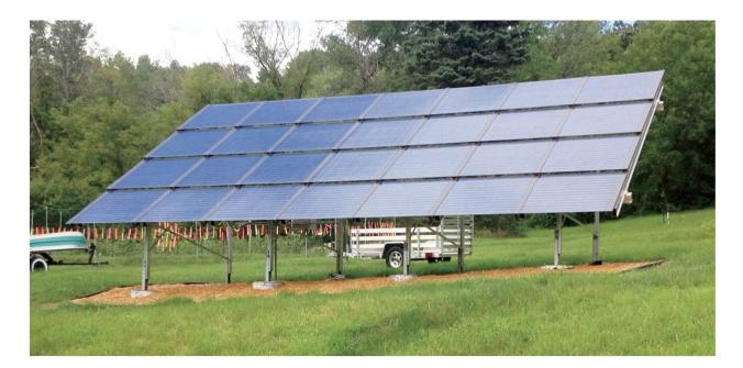
ABOVE: Ground-mounts can be located and positioned for optimal sun exposure.
