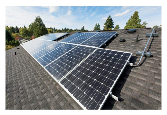
ABOVE: Conduit mounts with elevated anchors and flashing ensure a watertight installation and provide for cooling airflow underneath the conduit, similar to that underneath the PV modules themselves.
