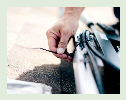
ABOVE: Plastic wire ties can wrap all the way around rails and are handy for tying up coils of wire.
