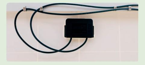
ABOVE: Wire clips for module frames help tame long module leads. These are usually metal or plastic, 1/4 inch in size.
