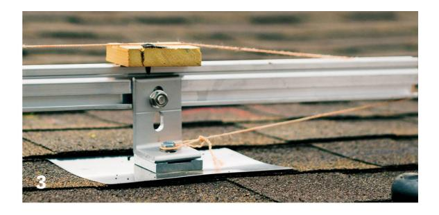
4. **Straighten the rail.** Working from one end to the other, measure between the string line and the top of the rail. Adjust the rail height at each footer so the rail is <sup>3</sup>/<sub>4</sub> inch (or whatever your block thickness is) from the line, then tighten the rail mounting bolt to secure it to the footer, torquing the bolt as directed. Repeat at each footer until you reach the other end of the rail.
